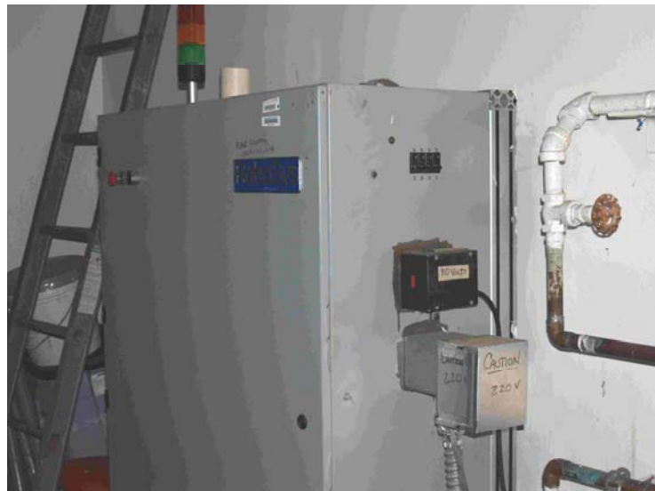
Figure 45 Filter Installation to Suppress Motor-Controller Noise
