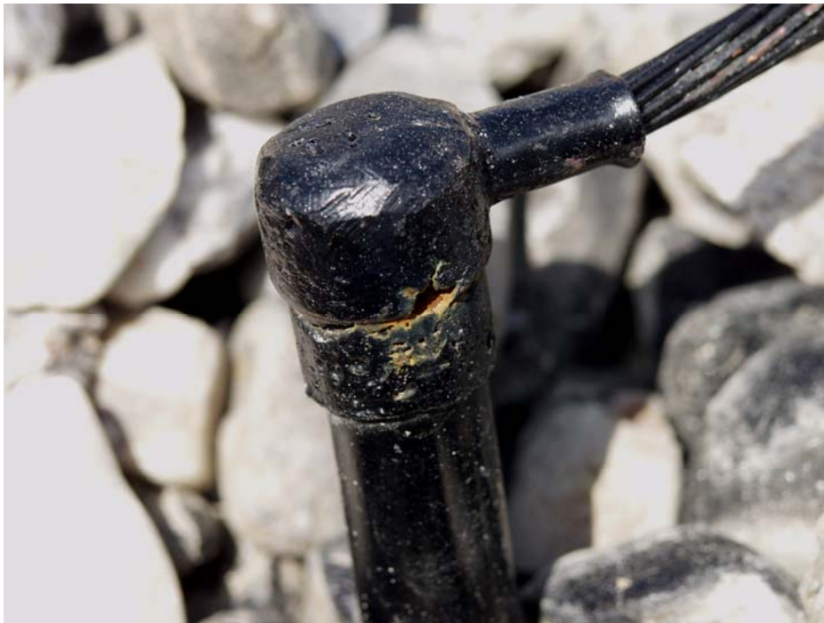
Figure 15 CADWELD® on Antenna Counterpoise Wire
