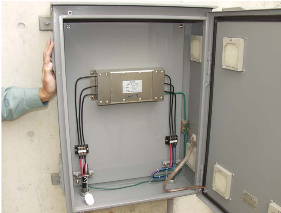
Figure 49 Improper Filter Configuration
