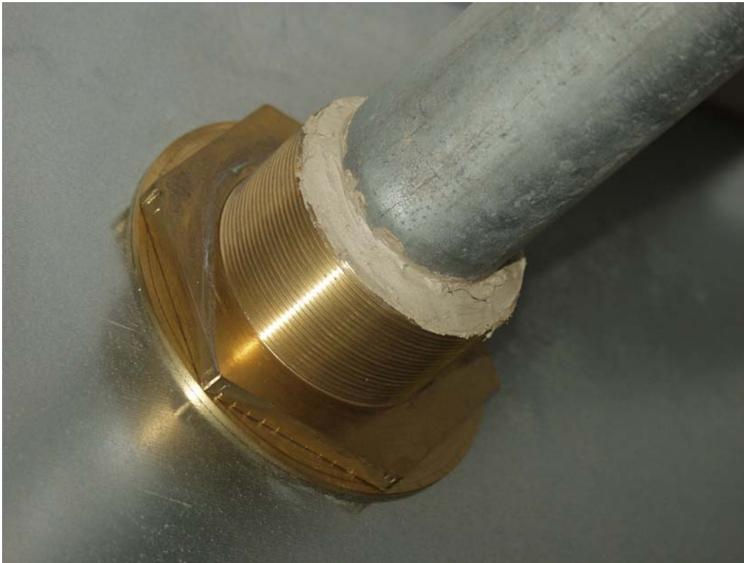
Figure 18 Water Pipe Penetrating a Shielded Room
